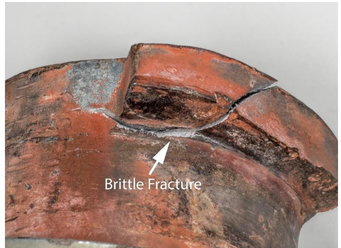
Figure 2 – Visual Indication of Brittle Fracture in Locking Clamp 1
